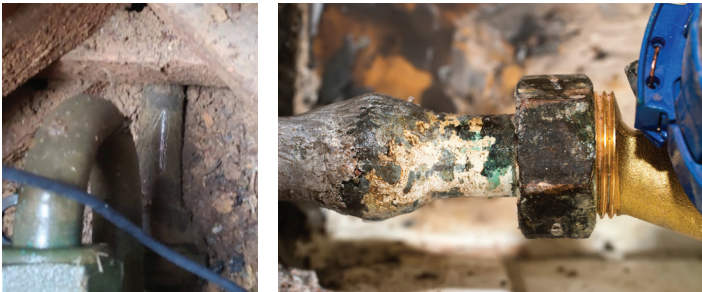
Lead pipes are wider at the base and can form a bulb.
